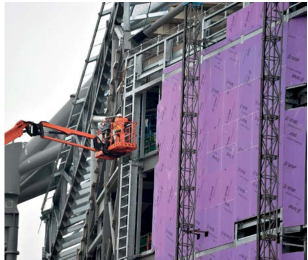
Gypsum sheathing has been widely used for many years in harsh overseas climates.
